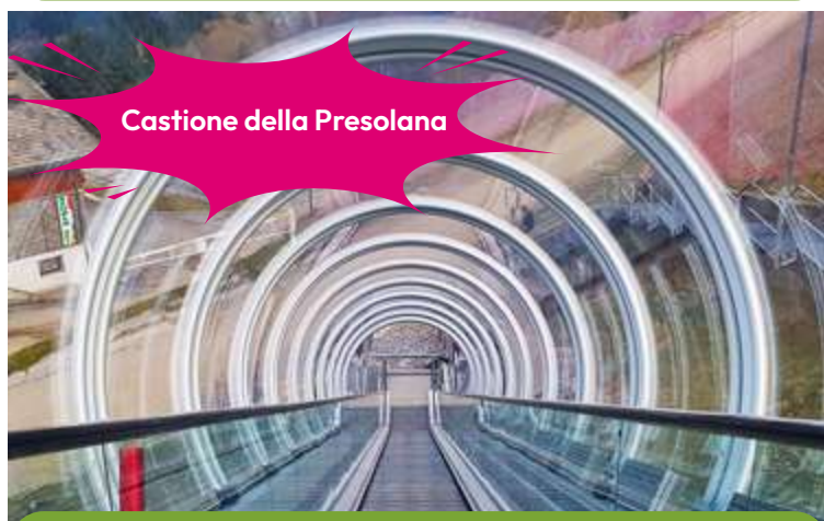
Copertura Scale Mobili Escalator coverage
